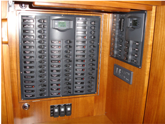
Hidden electrical panel
